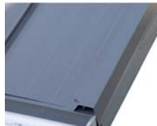
Fix the flashing No. 27. Don't forget the sealing compound.
