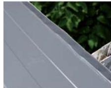
Bend the end sheet upwards.
