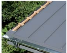
Trim the end sheet accordingly. Use a trimmer or similar to do so but never an angle grinder!
