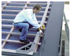
Lay the first sheet at right angles to the eaves.
