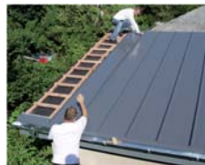
Large roof surfaces are covered very quickly.
