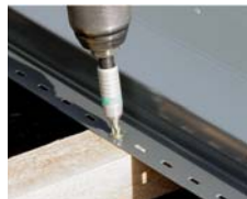
Fix the elements on the sub-structure using the Clip Fix screws provided.
